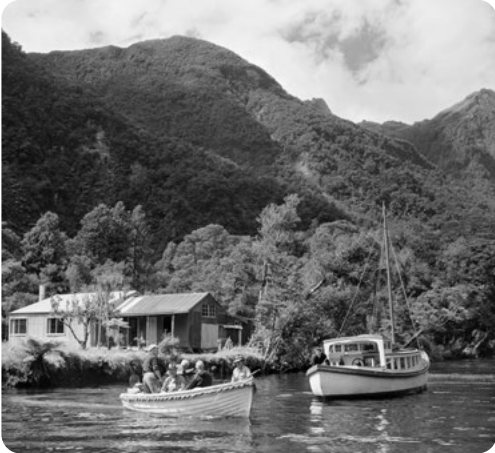
The Lyvia Lodge on the banks of the Lyvia River, Deep Cove, 1955. ALEXANDER TURNBULL LIBRARY. F-30660-1/2
